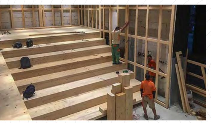
The Children's Playground Project in Istanbul Beylikdüzü Cultural Center has been completed. The project, which was built as an indoor playground and library, was manufactured using structural laminated wood and structural cross laminated wood (CLT) materials. The project, which was completed with non-toxic paints and varnishes in order not to harm health, started its activities in 2018.
