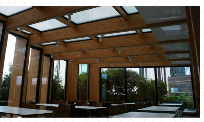
Two different structures which were planned as a winter garden for showroom and a café and projected by Erginoğlu and Çalışlar Architecture, were built by using structural laminated wooden joists in the garden of Çanakkale Seramik Headqurters in Levent/Istanbul. It is a modern project created a cosy venue reflecting the warmth of wood and glass is enhanced in combination with the use of wooden.
