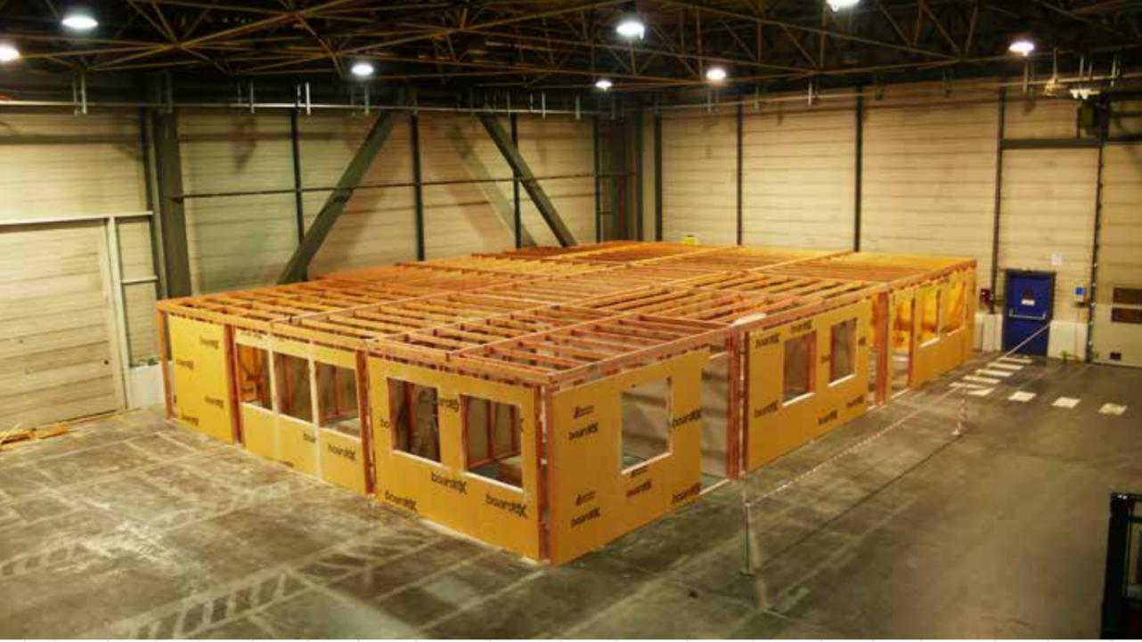
*It is the project of a single storey office located in Gölcük Ford Otosan's Supplier Park, SAS Automotive Production plant. Timber framed structure was built in accordance with the related regulation on an area consisting of 250 square meters.*
