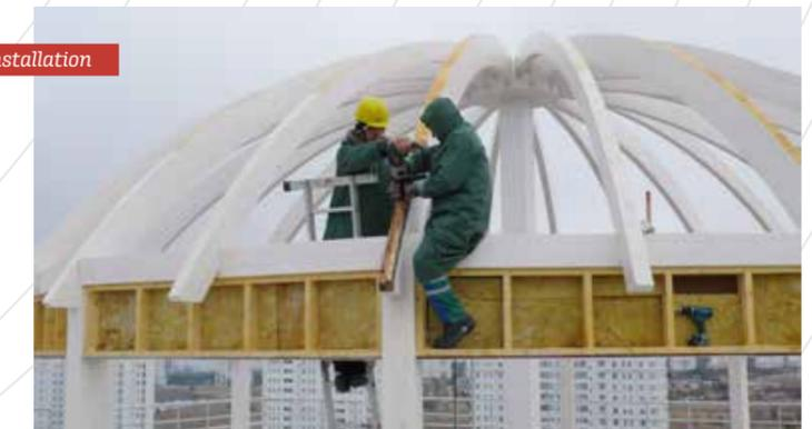
The structure having 12 m diameter is located on the terrace of Russia Federation Embassy -13storey building in the capital city Ashgabat. Without using a metal connection technology product, it was built with wooden dowels and interlocking system by forming radius timber truss. The dome that was the highest building of Ashgabat stands out with its location, architecture and construction technique.
