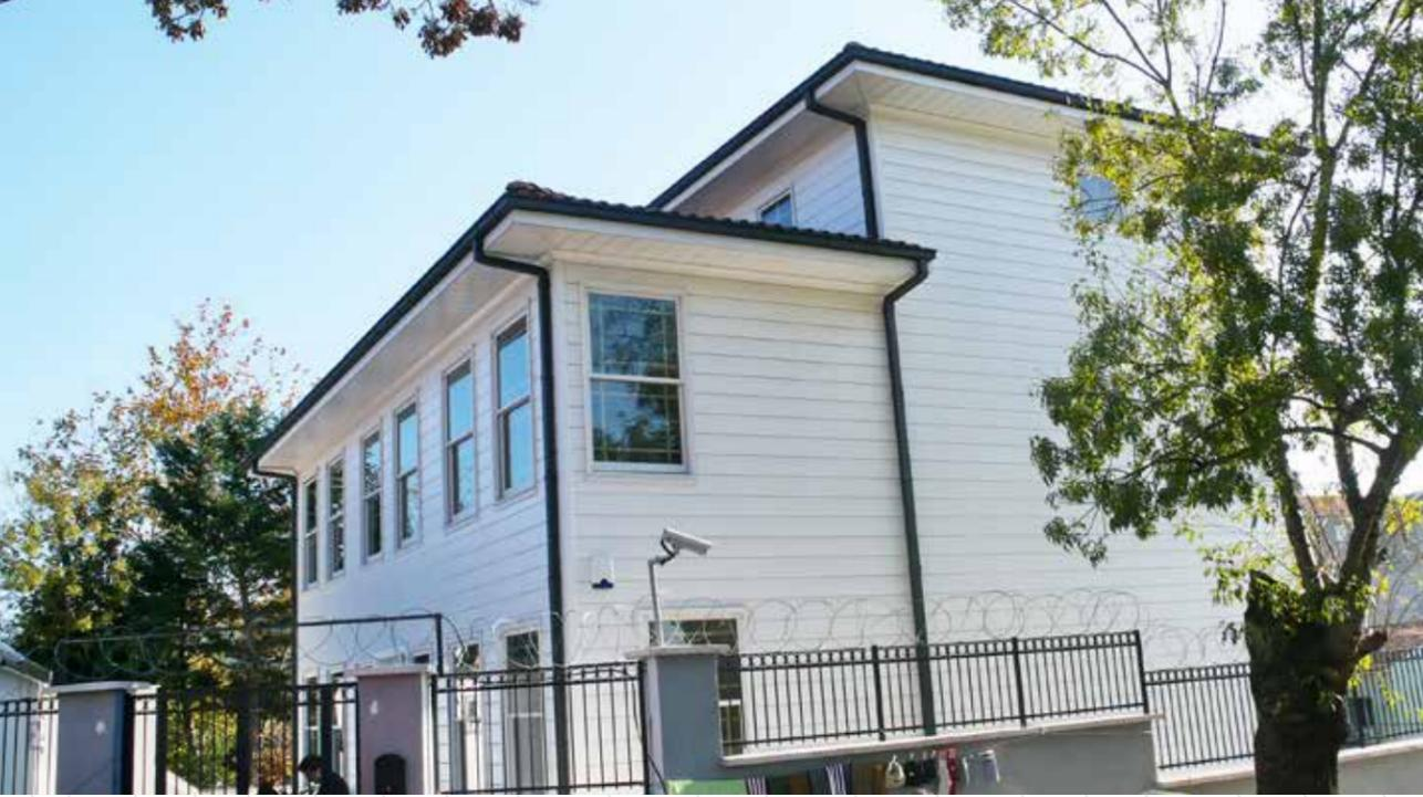
The building which was collapsed as a result of a fire in 1980's, was registered as a second degree historic building with the approval of The Council of Monuments. It was rebuilt with the wooden framework technique and now it is used for the commercial purpose.
