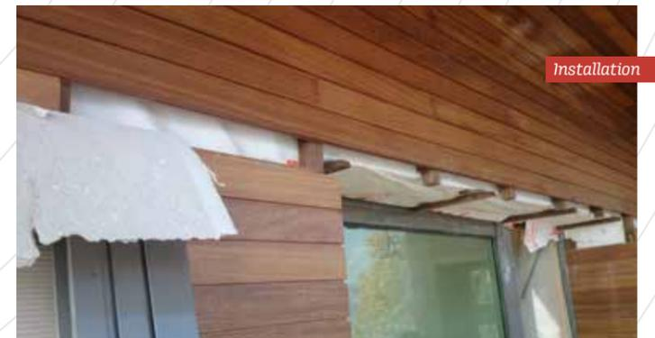
*Whole exterior curtain walls of this reinforced concrete structure in the most beautiful location of Emirgan, was made by using iroko thermowood process. It was a turn-key project and structural laminated wood materials were used as architectural elements of exterior walls of the building.*
