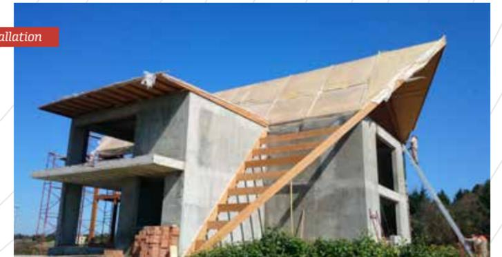
*It is a roof structure application for the reinforced concrete building located on a hill that dominates Terkoz Lake at Durusu Park. This roof structure with its steep roof form that was built by using structural laminated timber roof trusses, has got a gothic cathedral shape; it is an example with its steep roof form which has not been built in Turkey before.*
