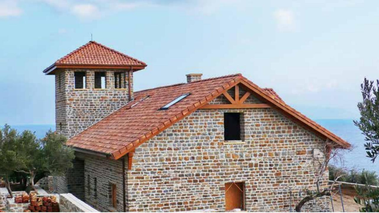
*It's built as a vineyard in Şarköy region famous for its vineyards, between Hoşköy and Mürefte with a view of Marmara island. The house was built with natural stones and it has a castle form with roof trusses using structural laminated wooden forms. The warm roof that covering the lounge where a fireplace is positioned with 360 degrees, is one of the most beautiful examples of stone and wood architecture combination.*
