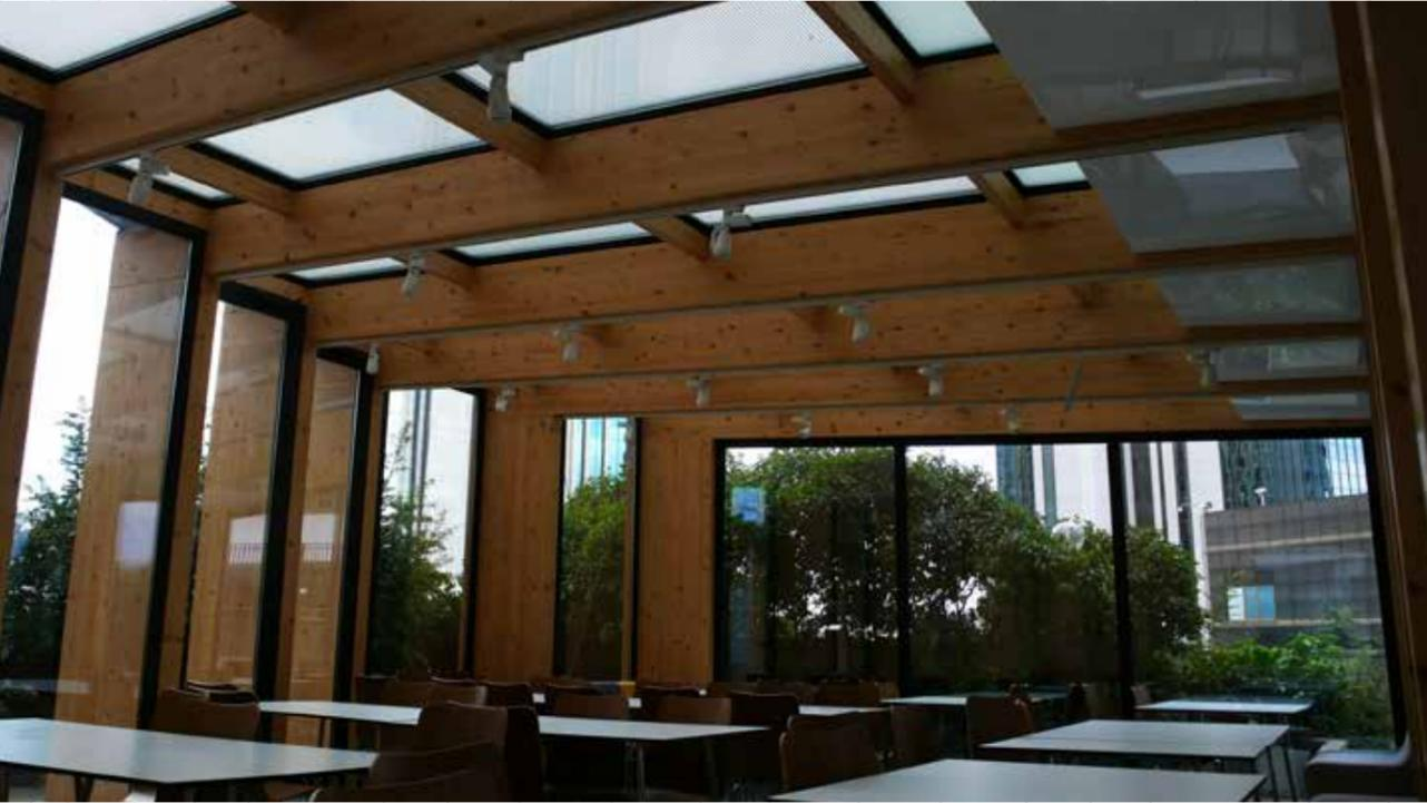
Two different structures which were planned as a winter garden for showroom and a café and projected by Erginoğlu and Çalışlar Architecture, were built by using structural laminated wooden joists in the garden of Çanakkale Seramik Headquarters in Levent/Istanbul. It is a modern project created a cosy venue reflecting the warmth of wood and glass is enhanced in combination with the use of wooden.
