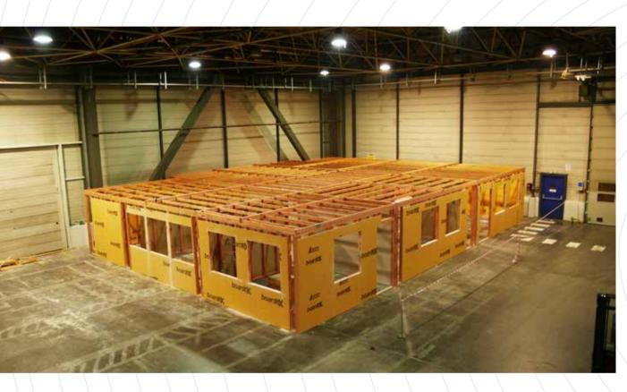
It is the project of a single storey office located in Gölcük Ford Otosan's Supplier Park, SAS Otomotive Production plant. Timber framed structure was built as fire-resistant building in accordance with the related regulation on an area consisting of 250 square meters.
